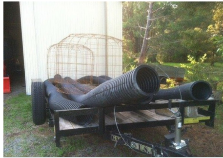
Constructed pond levelers ready for installation.
