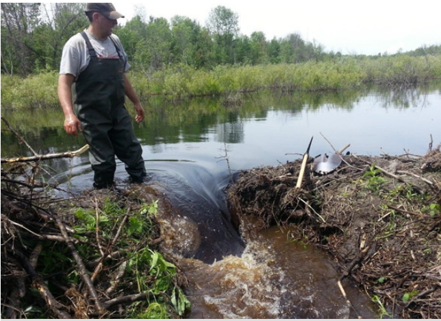
Breaching dam before installing pond leveler
